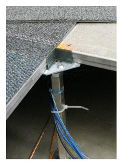
The bottom line is that, through all this work, the original carpet installer never had to return. Each trade that needed to access the floor plenum simply lifted the indicated carpet tiles, removed the floor panels underneath, then replaced panels and tiles when finished. None of these tradesmen had worked with the CarpetLOK system before, and they received no special instruction; it's that intuitive.
