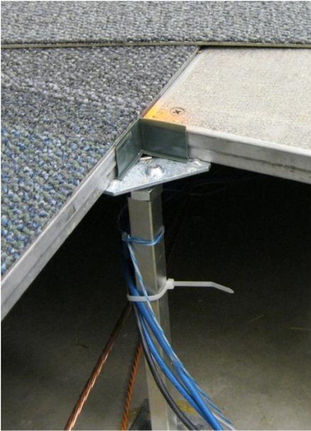
The bottom line is that, through all this work, the original carpet installer never had to return. Each trade that needed to access the floor plenum simply lifted the indicated carpet tiles, removed the floor panels underneath, then replaced panels and tiles when finished. None of these tradesmen had worked with the CarpetLOK system before, and they received no special instruction; it's that intuitive.
